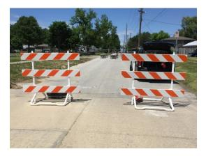
Where no turns are intended, the stripes should be positioned to slope downward toward the center of the barricade or barricades. *Opposite of above photograph*
